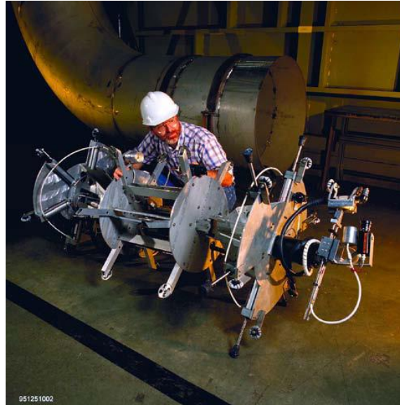
Pipe Inspection robot (Savannah River)
